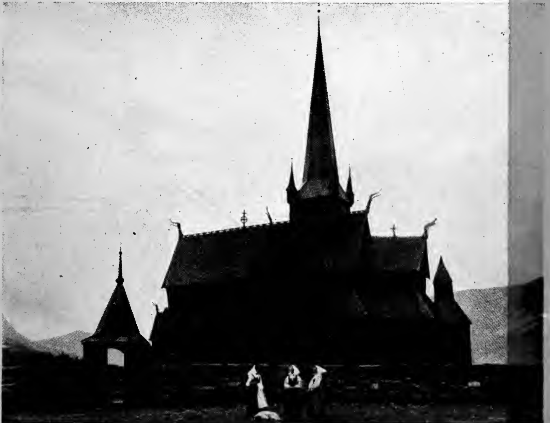
LOMS CHURCH. Part of it was erected 1115 A.D. It is renowned for its beautiful wood-carvings.
